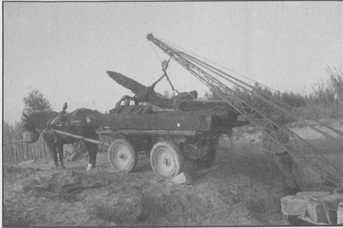
Fig. 3. Horse-drawn crane and wagon moving a timber. Photo courtesy INA Archives
